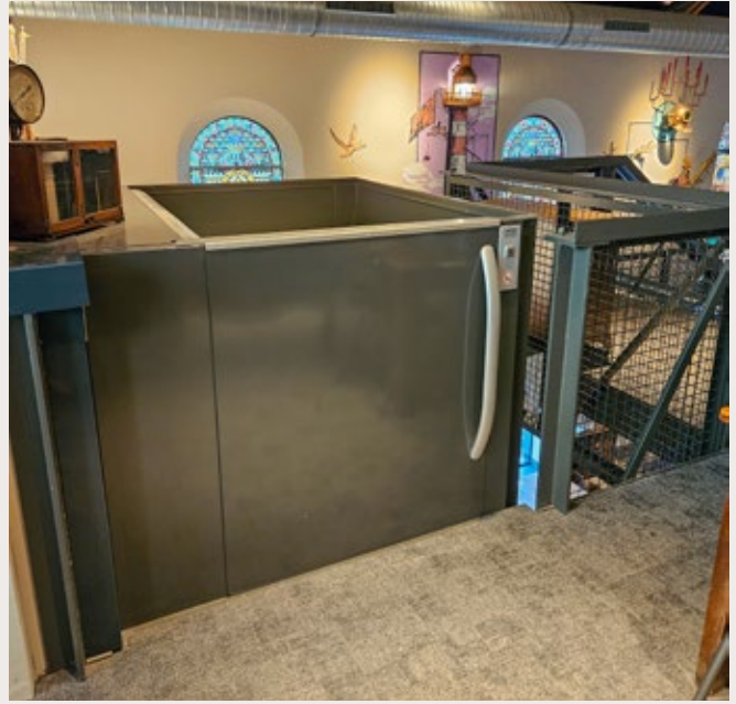
The lift has a 43 ¼" high gate on the top floor that makes the limited space of the mezzanine feel both open and airy.
