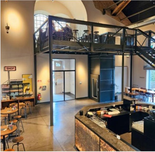
The resto-bar of the micro-brewery is equipped with a Cibes Primo platform lift to facilitate access to the mezzanine floor.
